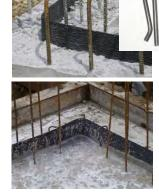
be fixed only by using the CEMflex clip. The overlapping has to be at least 5 cm; gluing the overlappings is not required!
